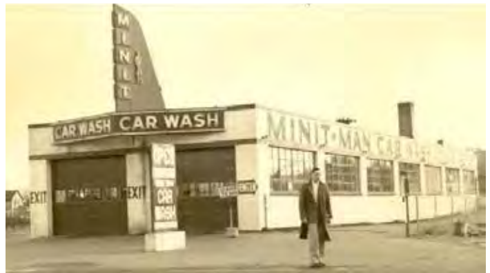
The current ScrubaDub in Quincy was once one of the historic Minit Man Car Washes.
