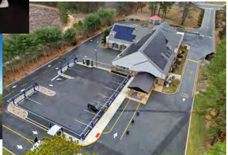
This aerial shot gives you a great perspective on the site's layout.
