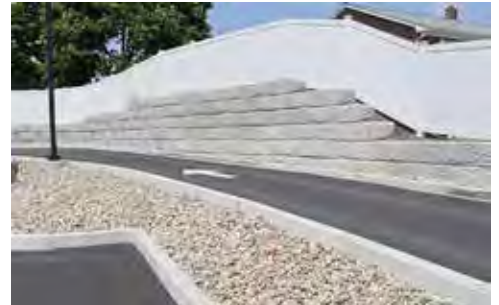
A great example of an effective retaining wall.
